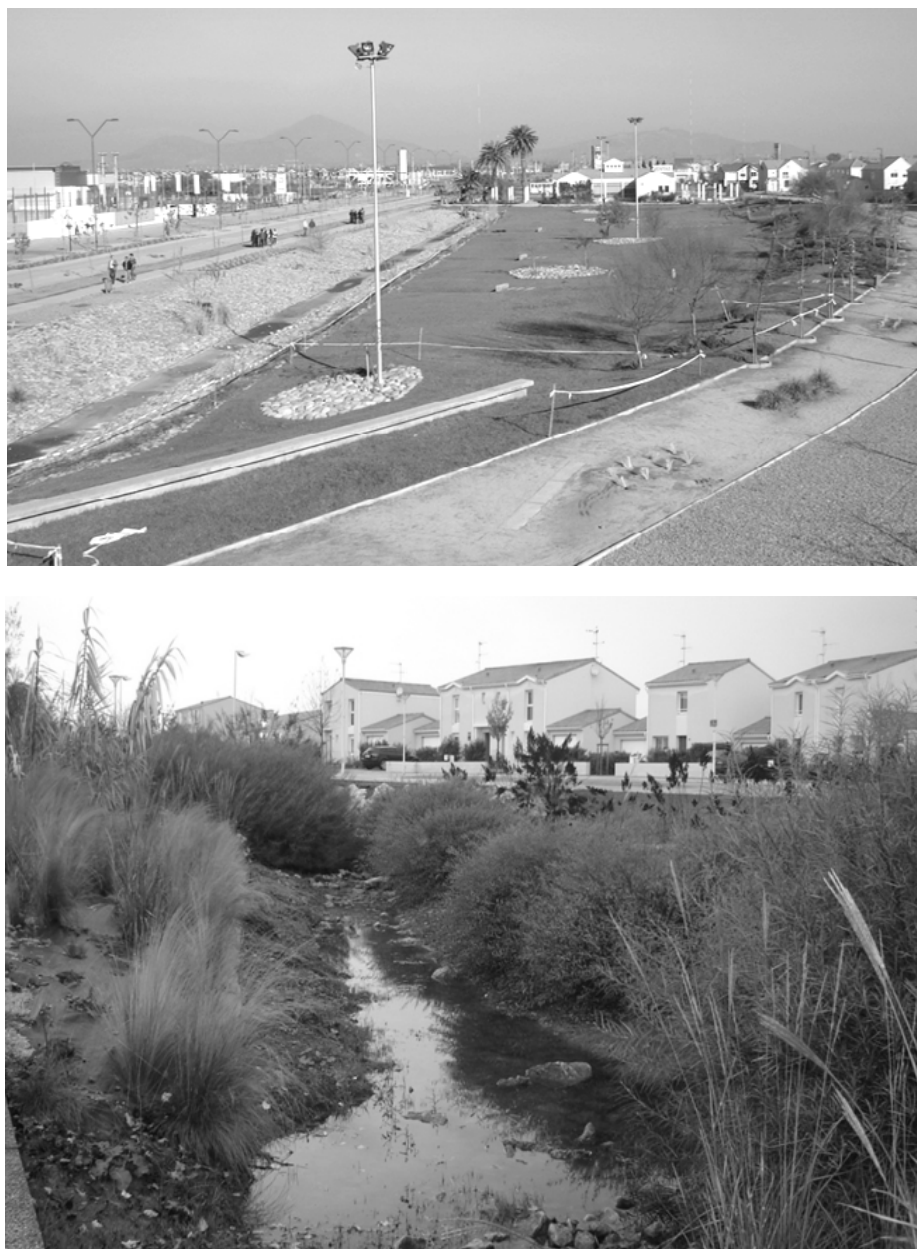
Figure 3: Examples of multifunctional landscapes – a detention basin in Santiago–Chile and a retention basin in La Rochelle-France. (Font: authors' personal collection, 2009).
