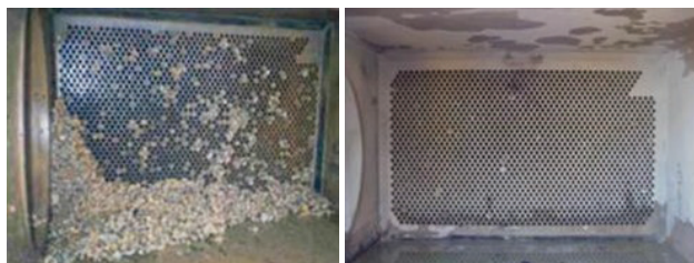
Figure 10. The effectiveness of the non-oxidizing biocide additive
